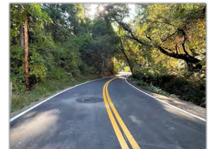
Smith Flat Road Project – New Pavement
