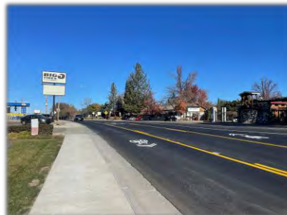
Placerville Drive Pedestrian Connectivity Project – New Pavement and Sidewalk
